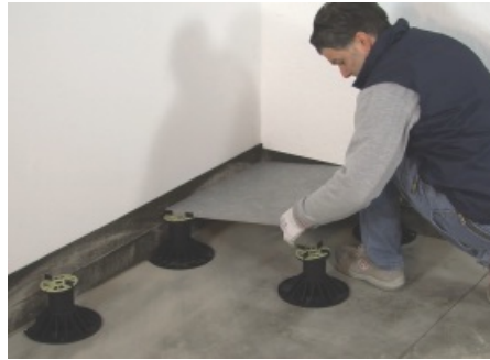
Adjust height with dedicated adjusting key
