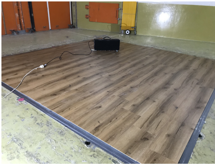
Figure 2.1: Flooring system installed on chamber floor
